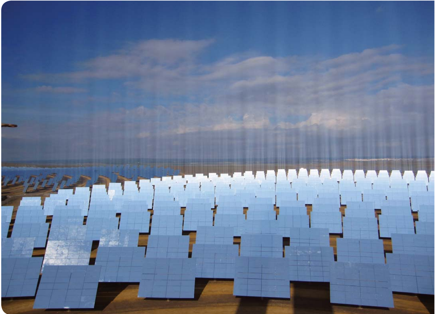
Solar power plant in Seville
